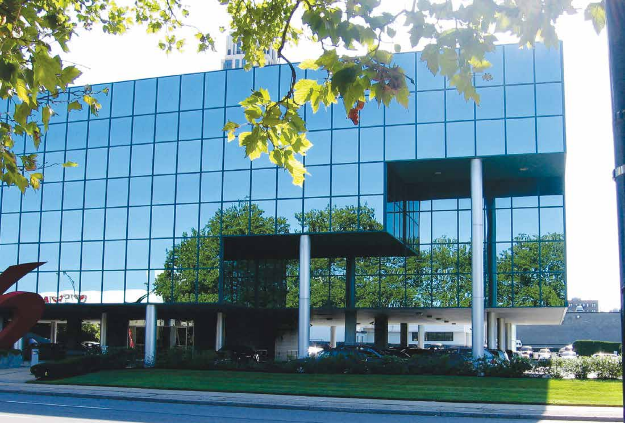
Mirrored glass is dangerous at all times of day, whether it reflects vegetation, sky, or simply open space through which a bird might try to fly. Photo by Christine Sheppard, ABC
