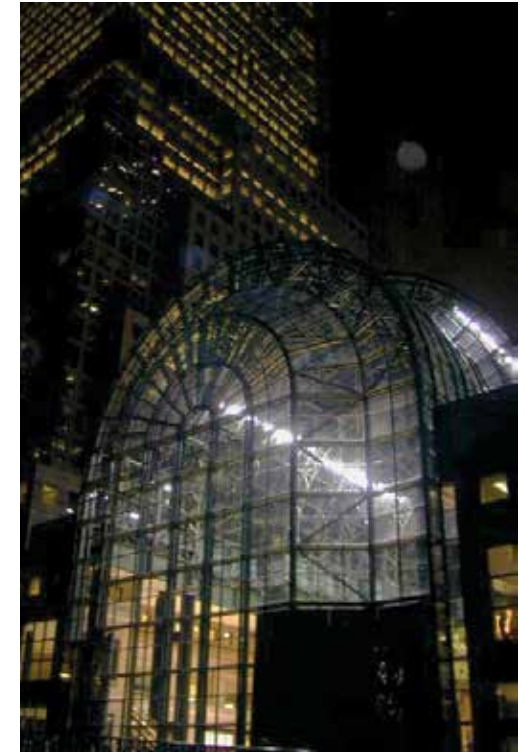
The glass walls of this atrium, coupled with nighttime illumination, create an extreme collision hazard for birds. Photo courtesy of New York City Audubon
