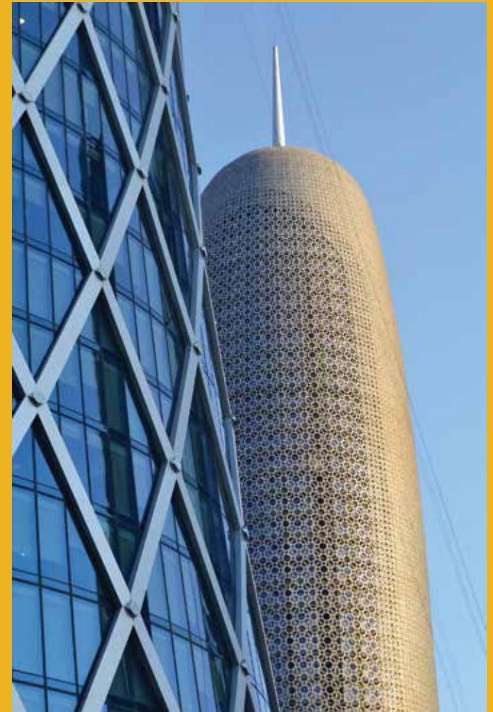
The Burj Qatar, designed by Jean Nouvel, was named Best Tall Building Worldwide in 2012. The façade, created with multi-layered screens, expresses local culture while providing protection from high temperatures and sand. Photo by Marc Desbordes
