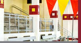
Interna-Rail<sup>®</sup> with Stainless Steel Wire Mesh Infill Panels
