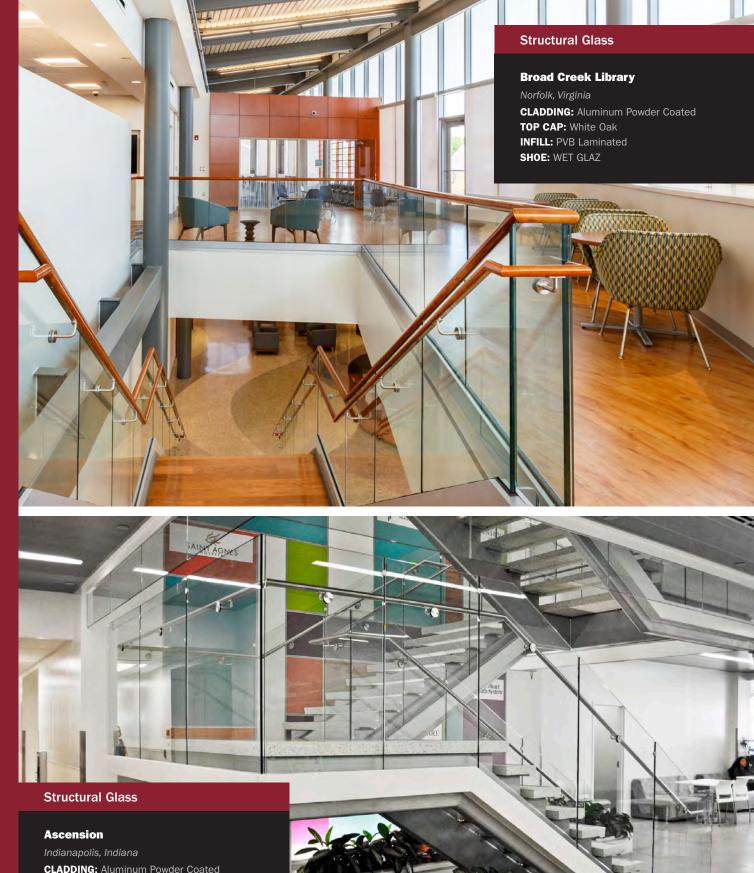
CLADDING: Aluminum Powder Coated TOP CAP: None INFILL: 1/2" Monolithic Glass
