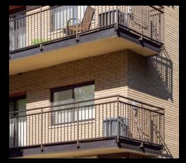
JP Management chose the Architectural Class 1 dark bronze anodized finish. JPM, O & S and Hollaender have found that this type of finish provides excellent protection against UV rays as well as being a more durable.
