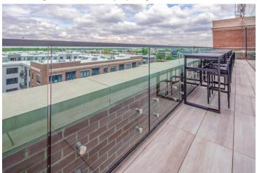
The buildings design incorporated outlook balcony areas with brick parapet walls, but they required guardrails in order for them to meet IBC guardrail codes. The architect team wanted to provide a safe rooftop environment and maintain the sweeping views, so Hollaender's Stainless Steel Button Mounts with 13/16" SGP glass and stainless steel U-channel top cap were specified and installed.
