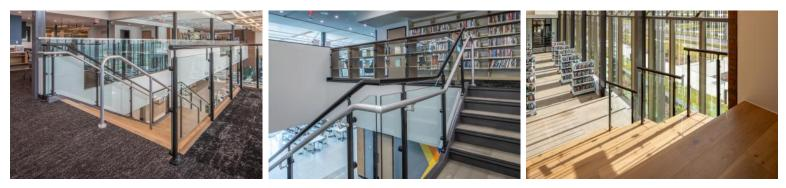
Hollaender also supplied structural glass railing systems for the interior overlook and outdoor patio. The use of anodized aluminum and glass railings creates an open, airy atmosphere while delivering safety, aesthetics, and cost-effectiveness, maximizing value for the community.
